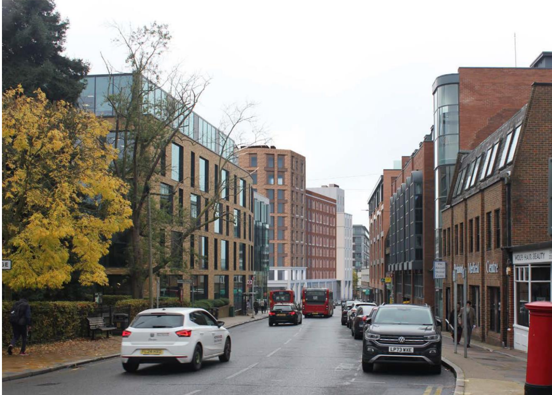
View of Proposed Development from Belmont Road towards High Street
