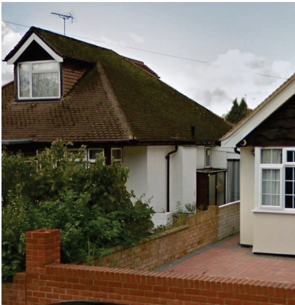
Figure 4 – October 2022 Street view imagery showing side structure in place at site
